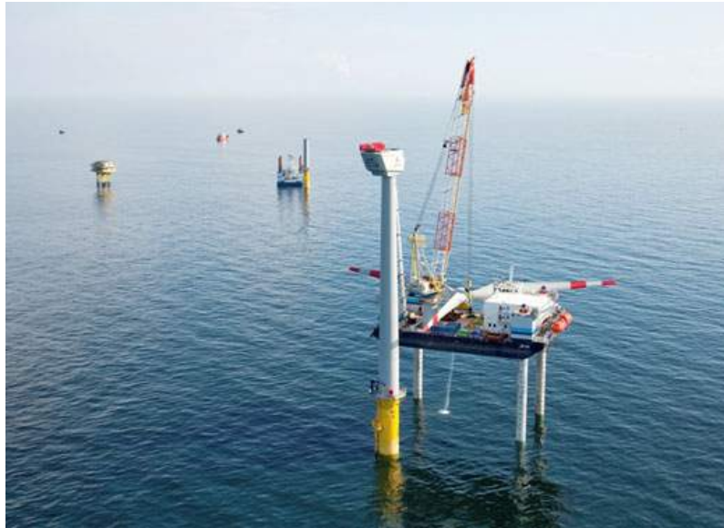
Figure 5.3: A jack up barge is used to replace or conduct maintenance on the rotor shaft or fan blades of a wind-turbine at sea.
